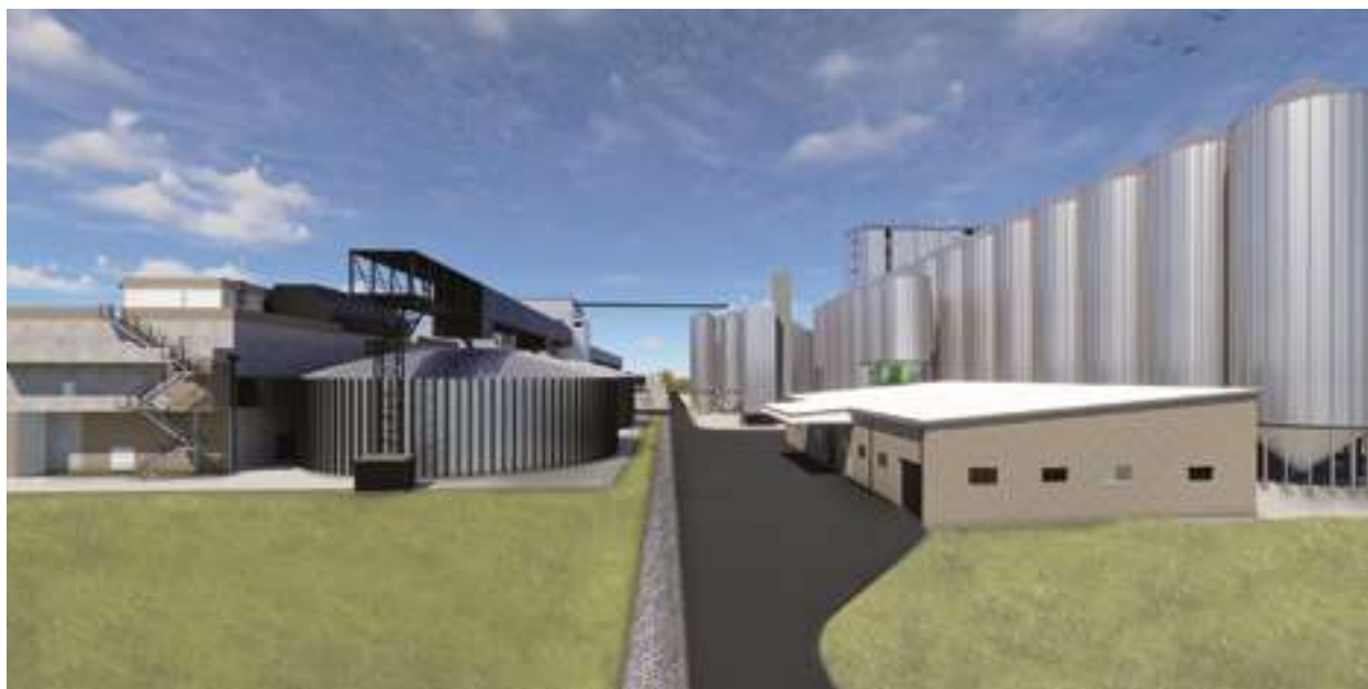
HEINEKEN and Soufflet Maltery Project
