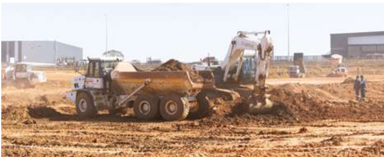
Precinct 2 bulk infrastructure development
